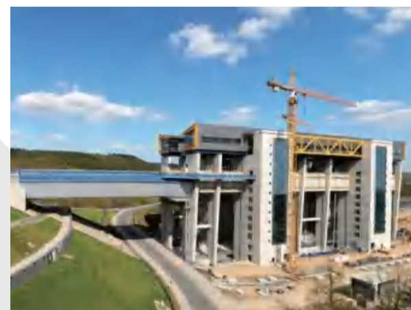
德国水工钢结构 Steel structure for navigation lock in Germany
