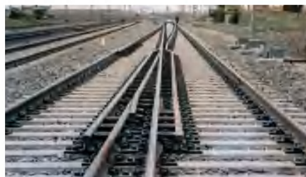
■ 时速250公里60kg/m钢轨38号可动心轨高速道岔 60kg/m No.38 movable-nose high-speed turnouts, Total length:136.2m, Straight speed:250km/h, Divergent speed:140km/h
