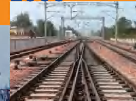
国内首组高速道岔研制成功，成功应用于秦沈客运专线 First set of high-speed railway turnouts in China, applied to the Qin-Shen Passenger Dedicated Line
