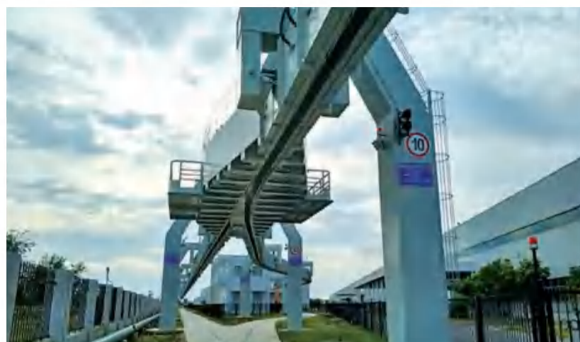
悬挂式空轨试验线 Suspension monorail test line
