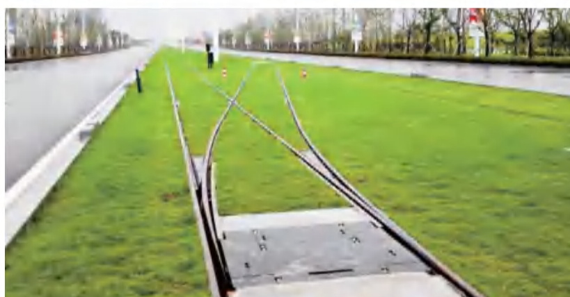
南京现代有轨电车59R2-6号单开道岔 59R2-6 Turnouts for Nanjing Modern Track transit
