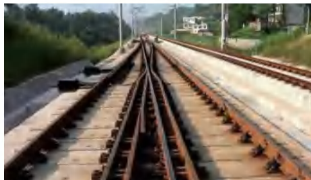
■ 遂渝线 (中国首条无砟试验段) Suiyu Line (China's first ballastless test line)
