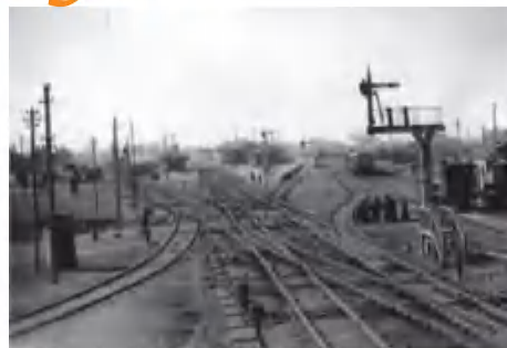
制造中国第一组铁路道岔 Manufacture of China's first Railway Turnouts
