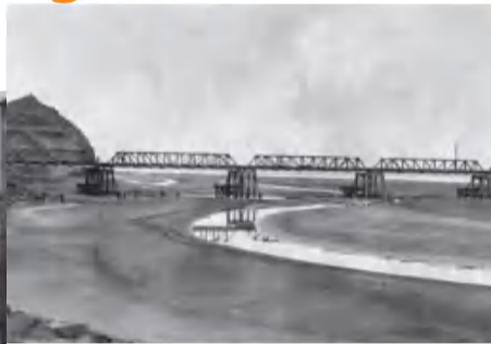
制造京汉铁路黄河大桥 Beijing-Wuhan Railway Yellow River Bridge
