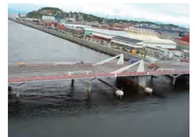
挪威尼德瓦开启桥 Moveable bridge in Nidvar, Norway
