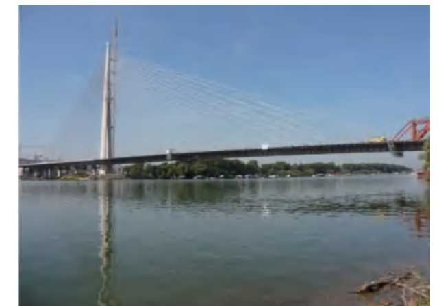
塞尔维亚萨瓦桥 Sava Bridge in Serbia
