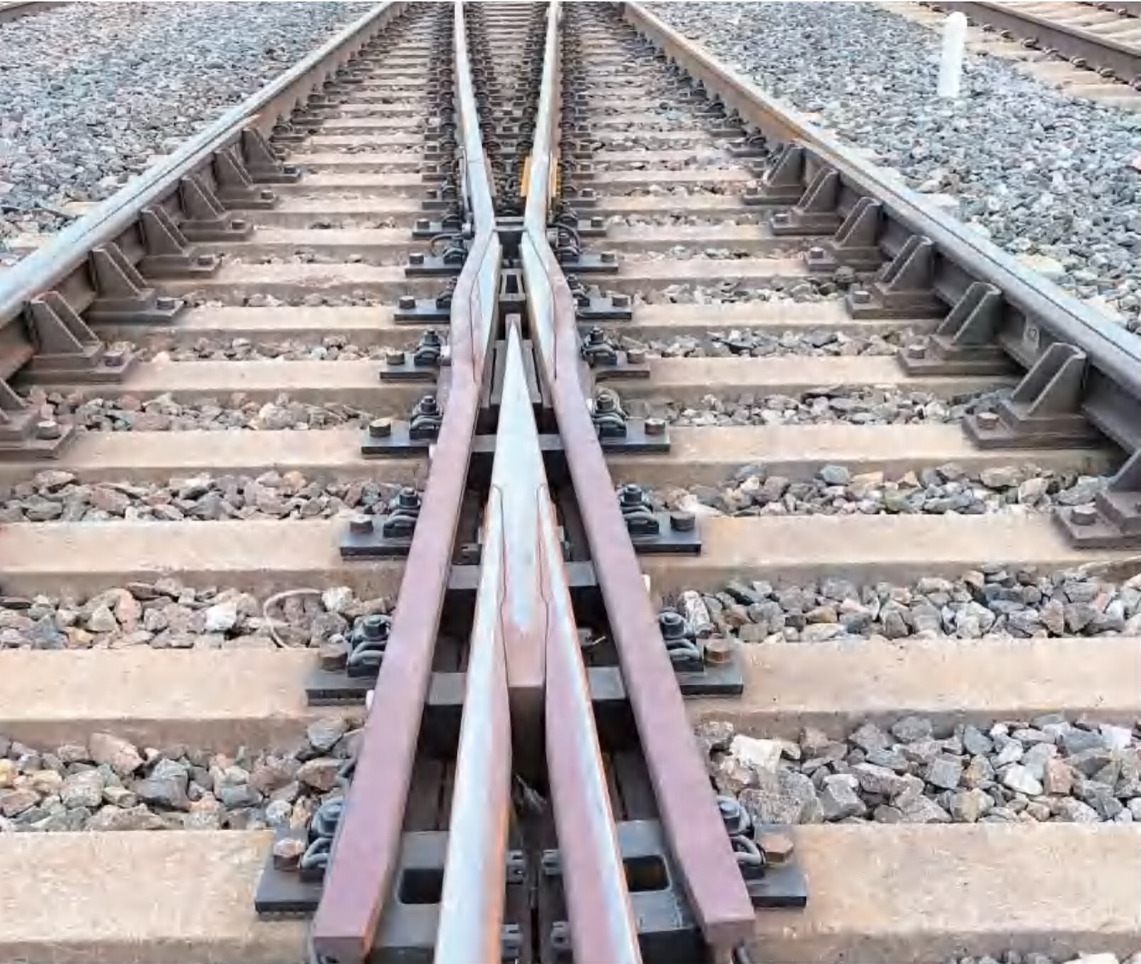
轧制高锰合金钢组合辙叉 Forged high manganese alloy steel combined frog
