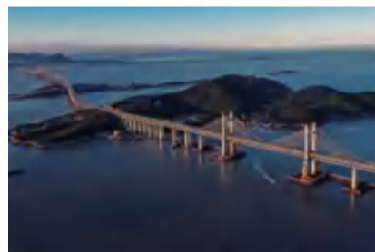
■ 福平铁路平潭海峡大桥 Fuzhou Pingtan Railway Pingtan Strait Bridge
