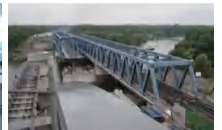
■ 德国双线铁路桥 Rathenow Bridge in Germany (double line railway bridge)
