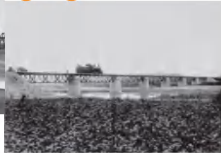
制造京张铁路全线钢桥 Manufacture of Beijing-Zhangjiakou Railway steel bridges
