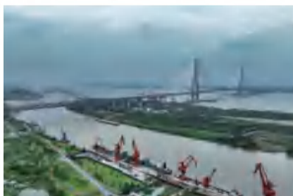
■ 常泰长江大桥 Changzhou-Taixing Yangtze River Bridge
