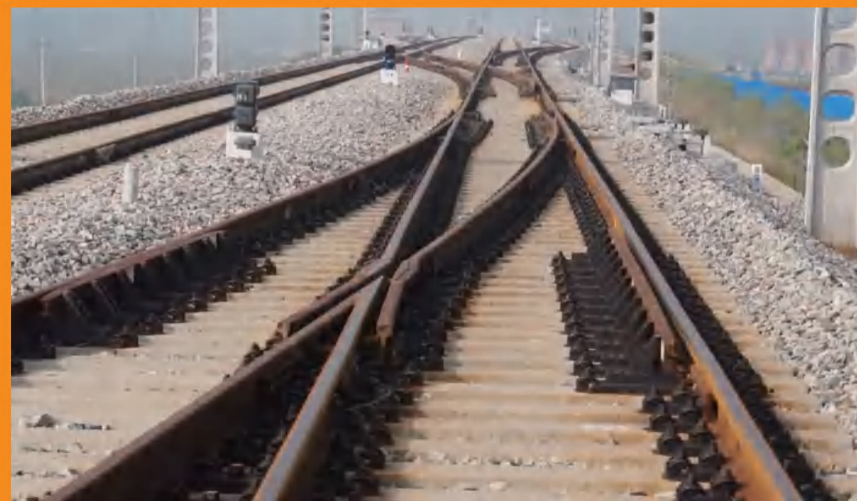
■ 30吨轴重75kg/m钢轨12号单开道岔 75kg/m rail profile, No.12 simple turnouts for 30 tons axle load
