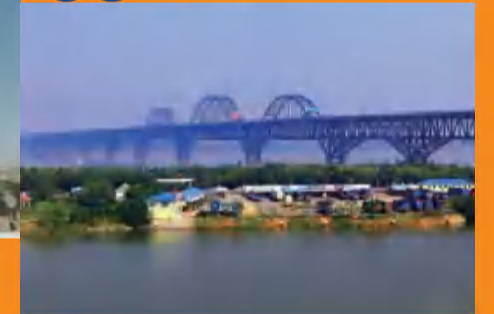
制造九江长江大桥 Manufacture of Jiujiang Yangtze River Bridge
